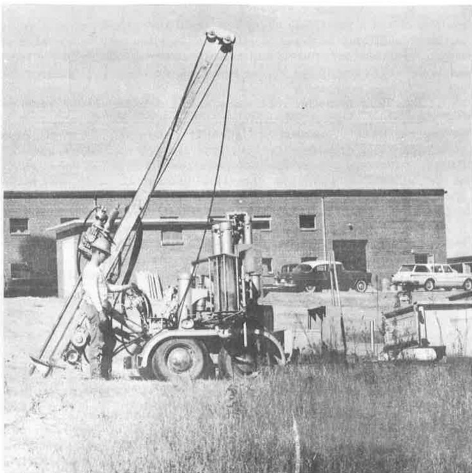
Figure 3. Vacuum-type drill rig used in geological investigation.
